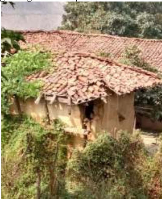
Figure 33 Household in lat which has been destroyed due to blasting in the Chhal Open Cast Coal Mine
