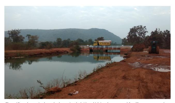
Figure 13: trucks carrying heavy loads crossing the bridge which is only constructed for villagers to cross and does not have the capacity to take 300 heavy loaded trucks every day
